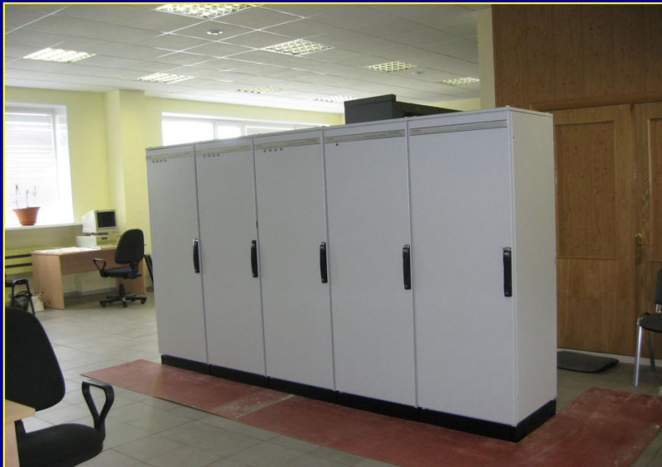
ASCS-12R' system boxes assembled in the main control room.
