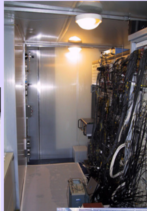
view with shielding completed
