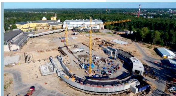
The construction site of the NICA complex
