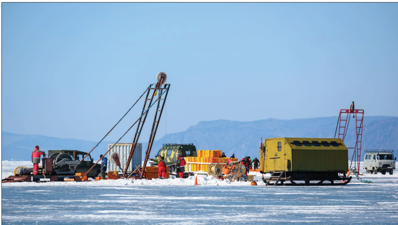
Baikal, March. Working moments of the expedition to build the deep underwater neutrino telescope Baikal-GVD
