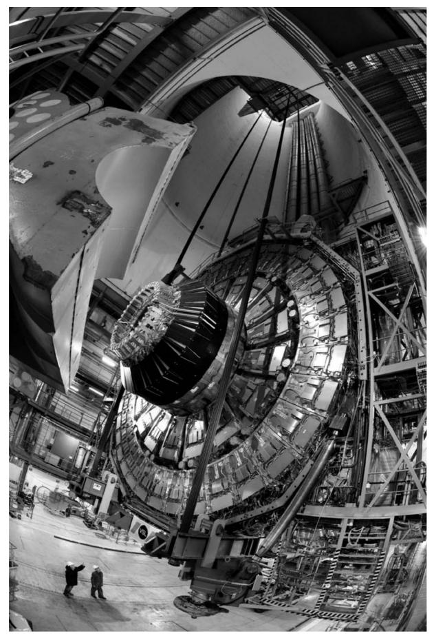
CERN (Geneva), 9 January. The YE+1 disk with JINR detectors is landing into underground experimental CMS hall to a depth of 80 m
