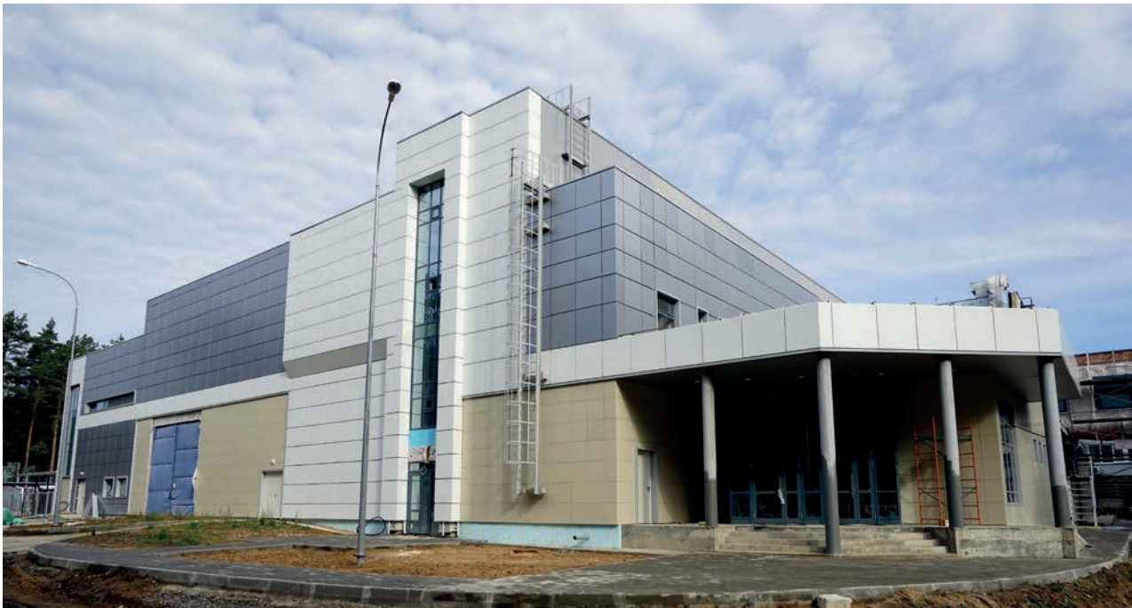
The Flerov Laboratory of Nuclear Reactions. The building of the Factory of Superheavy Elements
