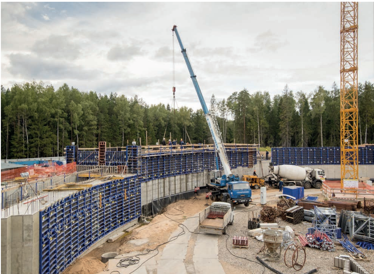
Construction of the NICA collider
