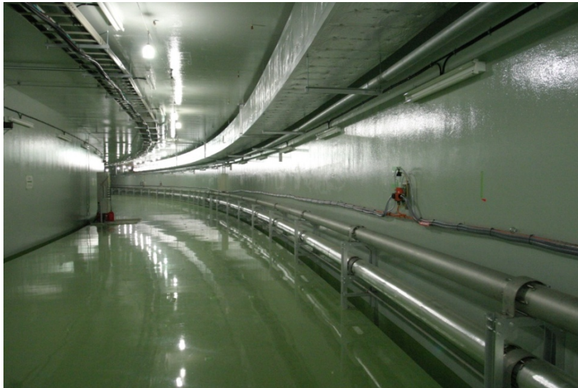
Level-measurement for the primary tunnel been done.
